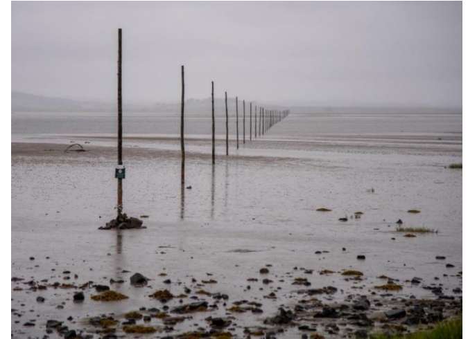
Above: the enigmatic Lindisfarne causeway Below: Telford's Menai Suspension Bridge in North Wales with Snowdonia in the background.
